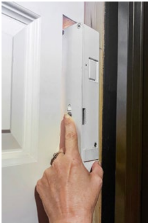
Insert at a downward angle
